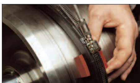
Stage 3: Clamp in position with steel band.
