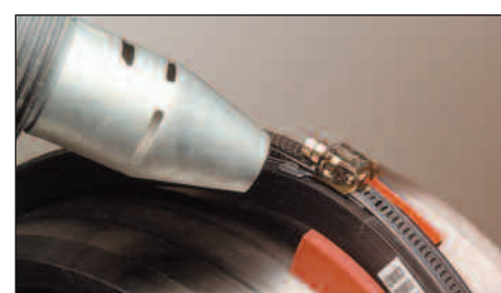
Stage 4: Cure epoxy adhesive with hot air gun.
